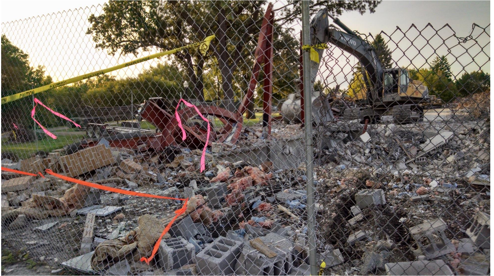
Digging out the crawl space cement
